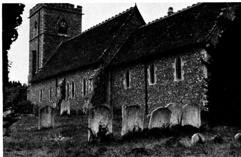
The third picture shows Buckler's drawing of the other side of the church, almost entirely old, picturesque and attractive. The fourth picture shows the same side but the church almost rebuilt.
